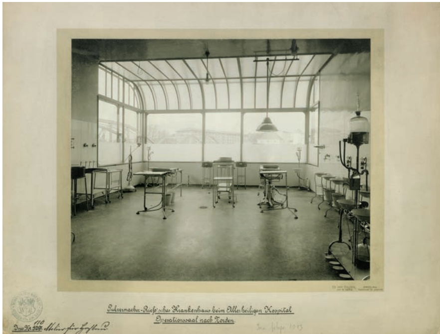
Wrocław, All Saints Municipal Hospital, operating theatre
